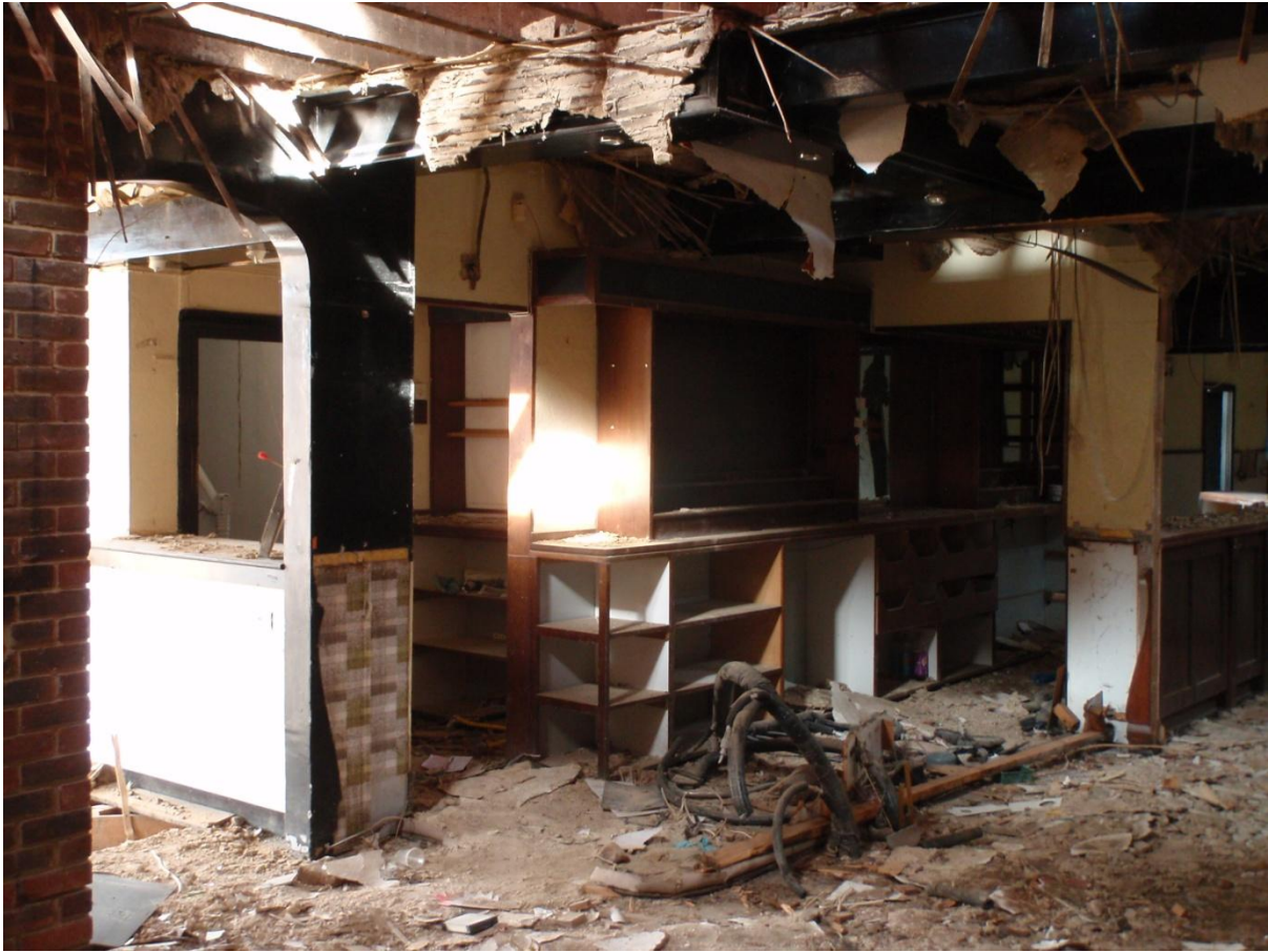
Plate 5. Interior view of the main front bar
