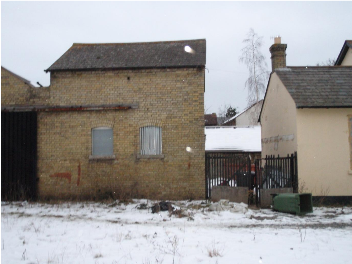
Plate 3. The rear of the Walnut Tree public house facing north east
