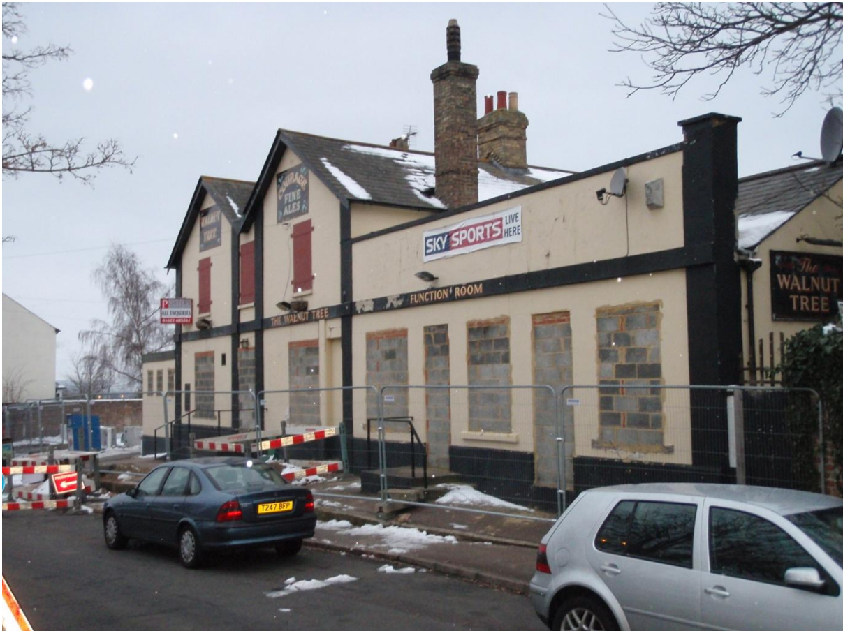
Plate 2. General view of site prior to demolition facing south west
